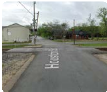
Absence of safe railroad crossings
