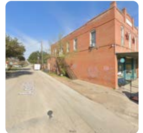
OC6: Flooding of local stores at the north west corner of Main and Ash Street - partly executed.
