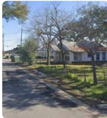
Drainage issues on the street
