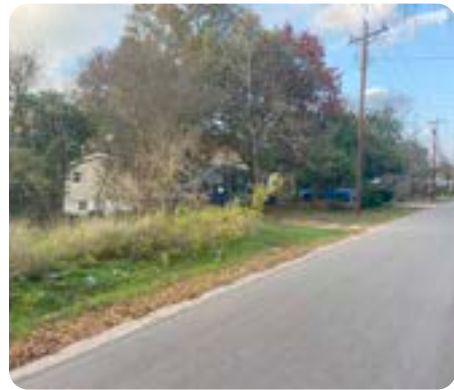
Absence of sidewalks
