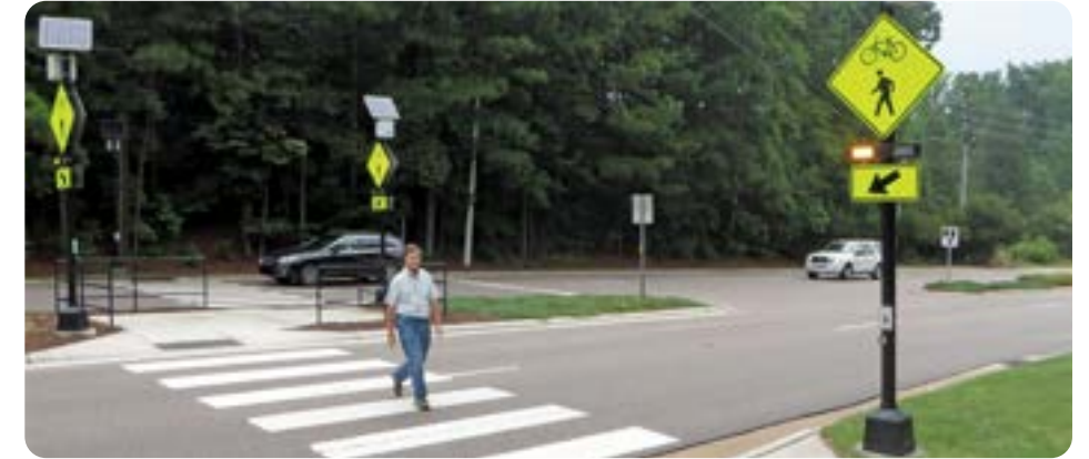
Pedestrian beacons can be used where traffic lights or stop signs are not present.
