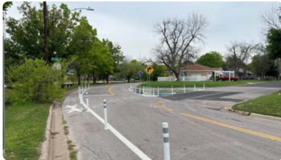
Painted tactical sidewalks and pedestrian refuge islands
