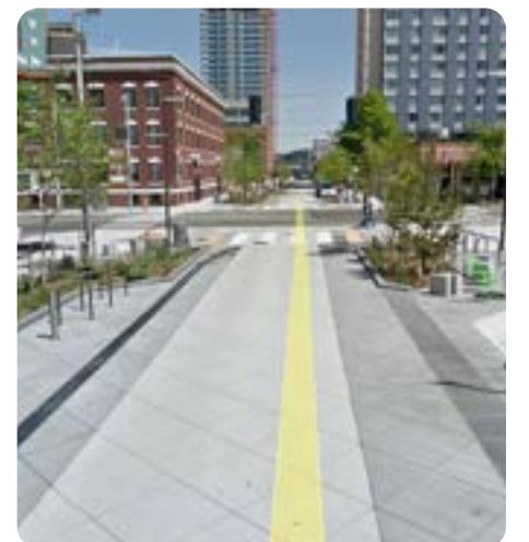
French drains and colored concrete is used in place of typical curb and gutter.
