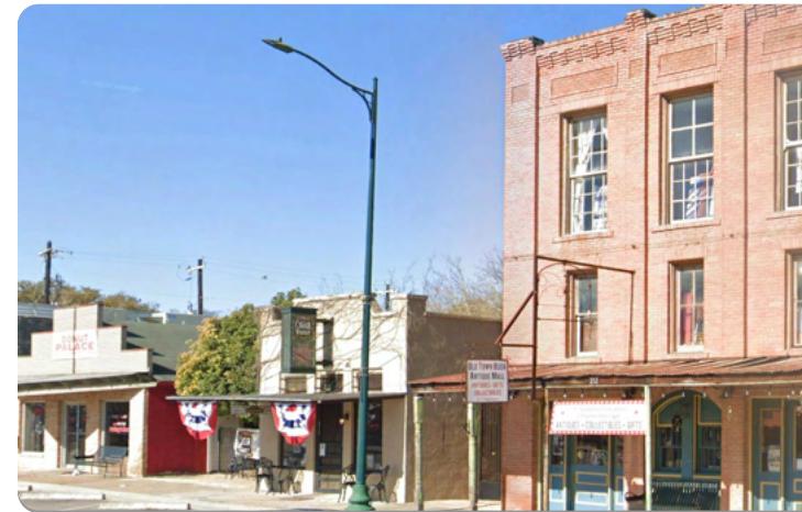
Existing Vehicular Lighting - Main Street, Buda
