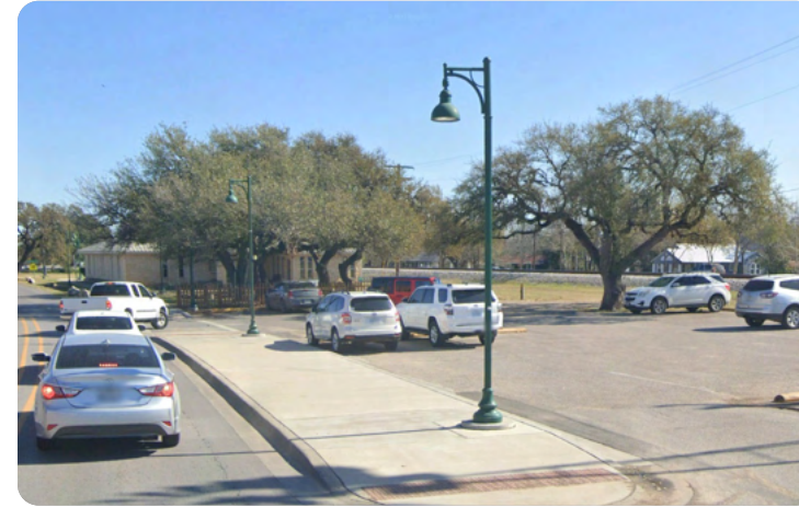
Existing Pedestrian Lighting - Main Street, Buda
