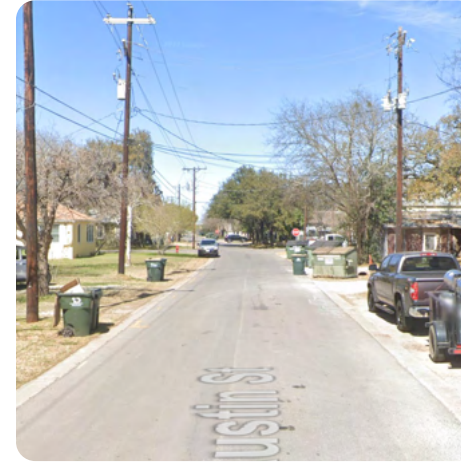
Power lines and residential properties
