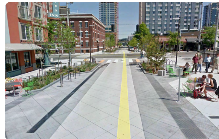
French drains and colored concrete is used in place of typical curb and gutter.
