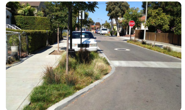
Shared Streets with laydown curbs provide spaces for water quality within the street, along with narrow travel lanes and signages.
